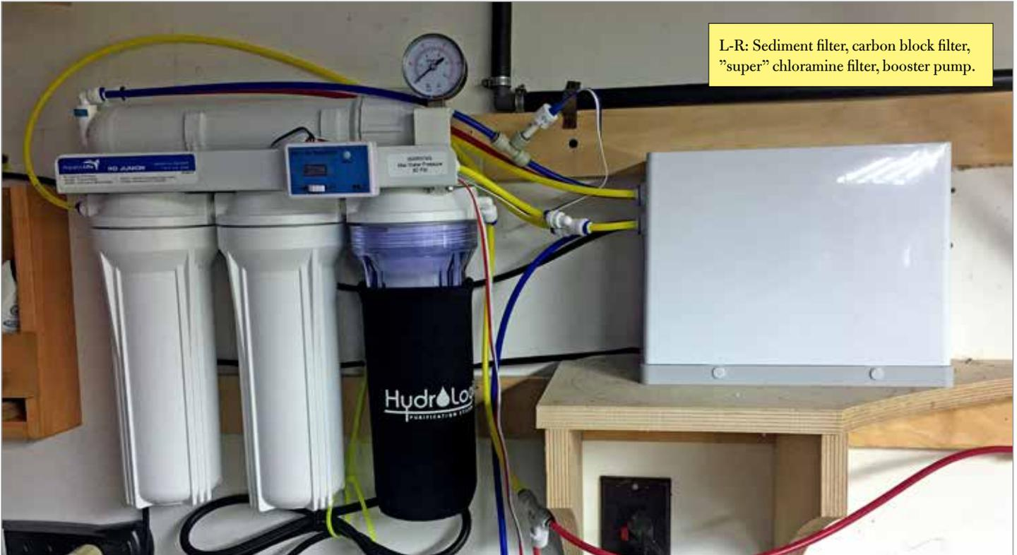
L-R: Sediment filter, carbon block filter, "super" chloramine filter, booster pump.
