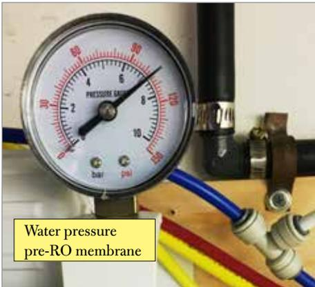
chain’s output directly to the membrane. Clean water runs into my 3-gallon output bucket, while the waste water goes out 20 feet or so via flexible 1/4-inch plastic pipe into my basement laundry tub, where it either is fed to a plastic 5-gallon storage jug, or is sent down the drain. I chose a 100 GPD (gallon-per-day) RO unit, as anything less capable takes too long to make clean water.
